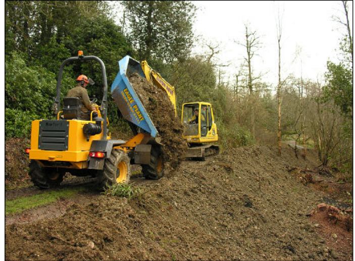
Building the Devon Hedgebank.
