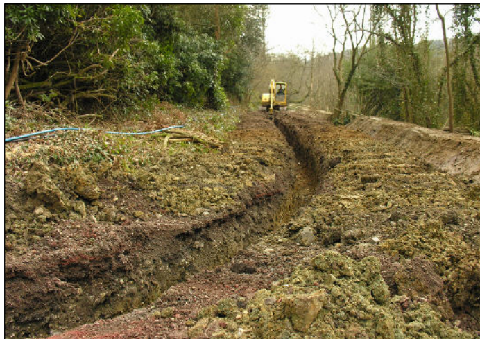
The new hedgebank and trench for water, power and data.
